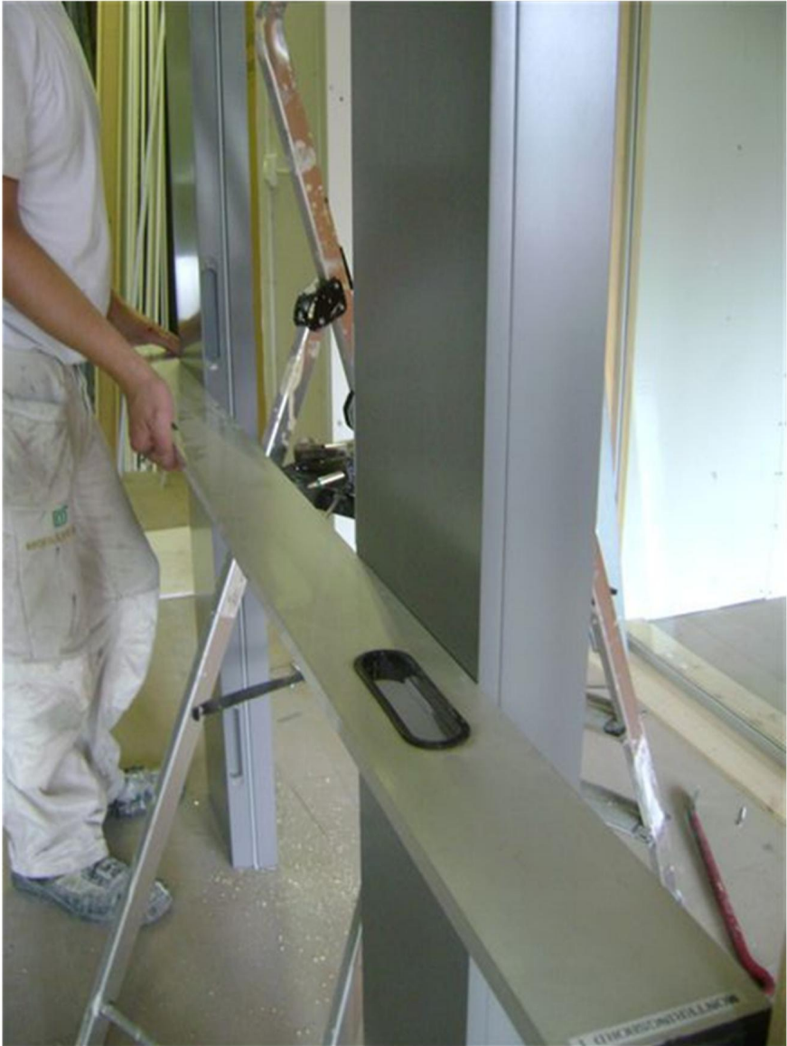
Adjusting side panels parallel
